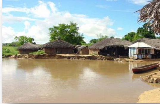
Figure 9: Houses in Rufiji Delta Built Using Mangrove Poles
